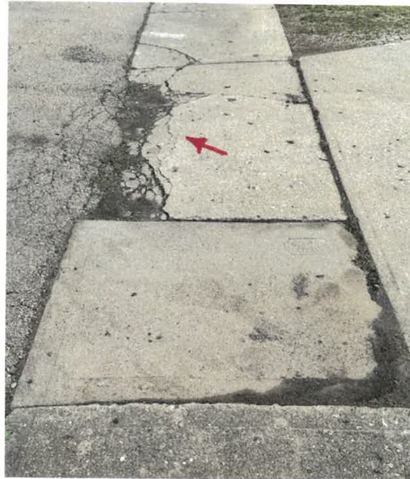
Sidewalk Cracking – Needing Replacement
