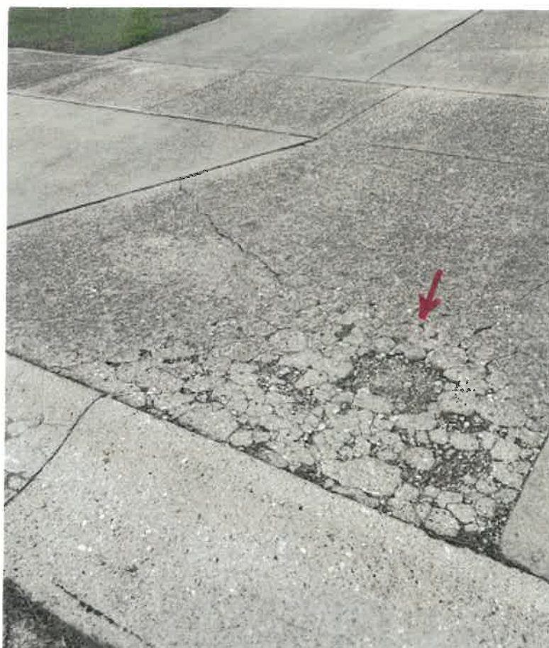
Drive Approach Cracking – Needing Replacement
