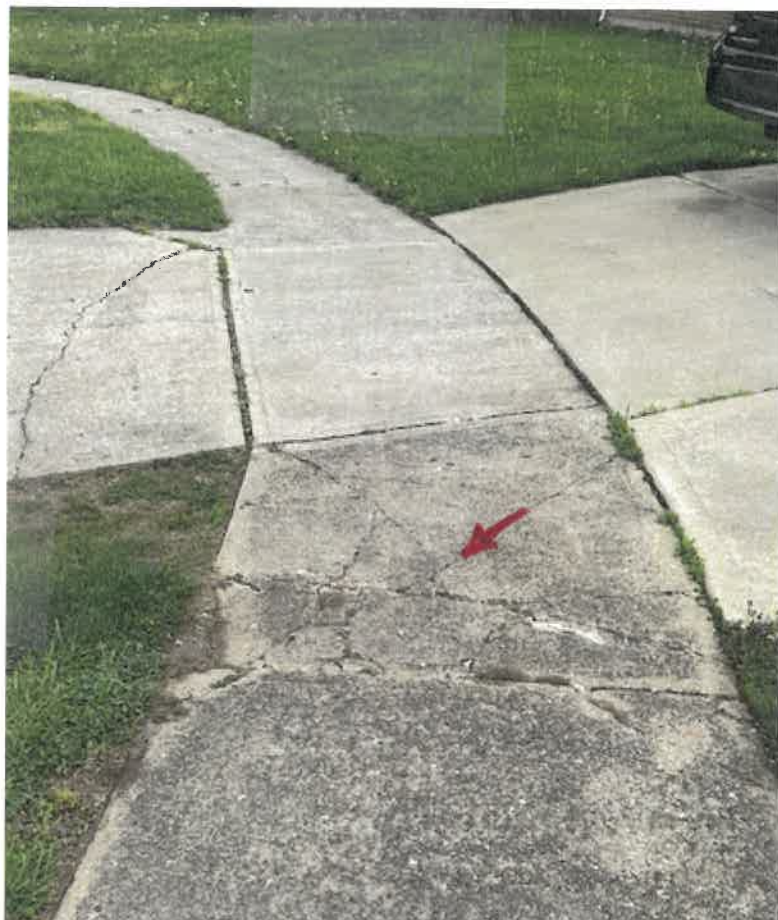
Sidewalk Cracking – Needing Replacement
