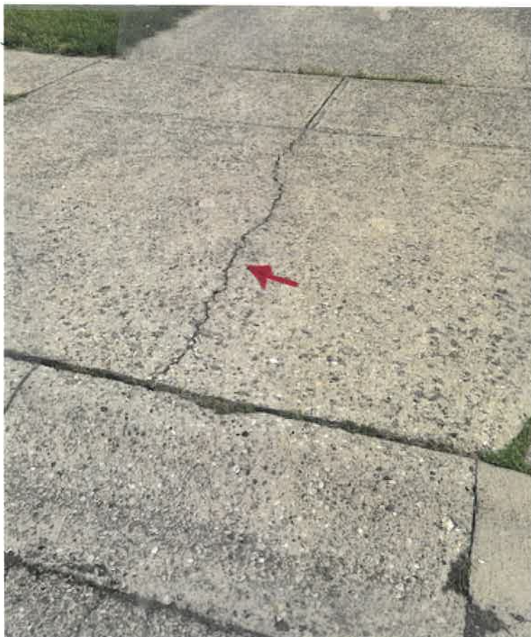
Drive Approach Cracking – Needing Replacement
